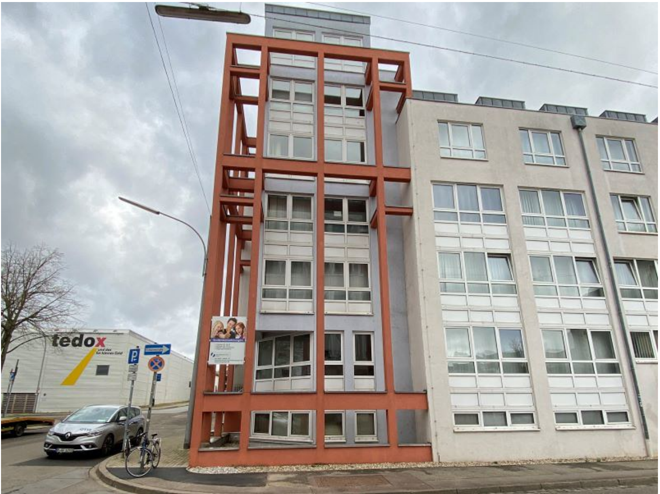
Exterior view dormitory Sulzbachstraße
